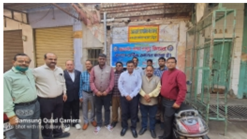
On the occasion of Children's Day, Alliance Club Hapur Crystal, District 142 installed an LED light at Adarsh Primary School for children..
